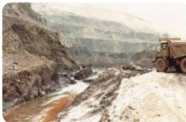
Photo 16. Trench digging for drainage and water conveyance to mine sumps. Source: MBR
