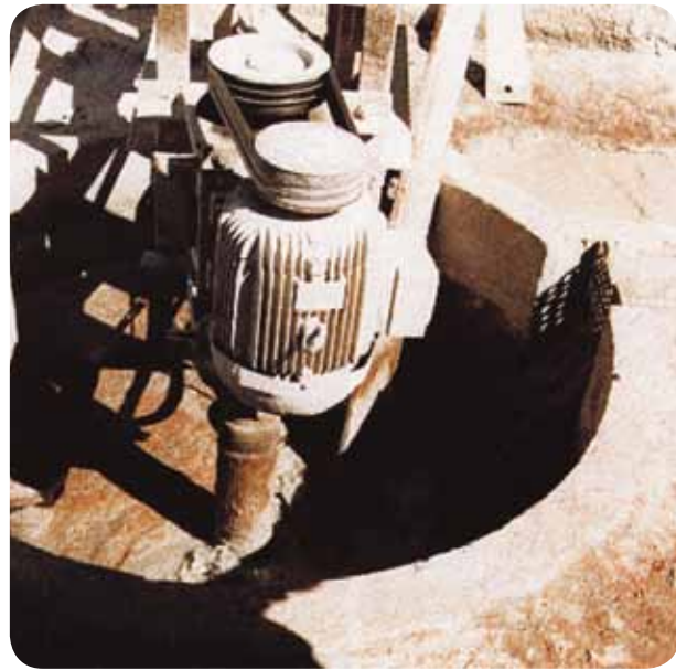
Photo 56. Waste pumping pit for final disposal
