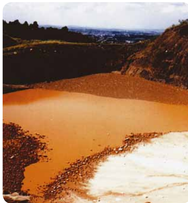
Photo 85. Sump and settling tank for rainwater, including sediments retained
