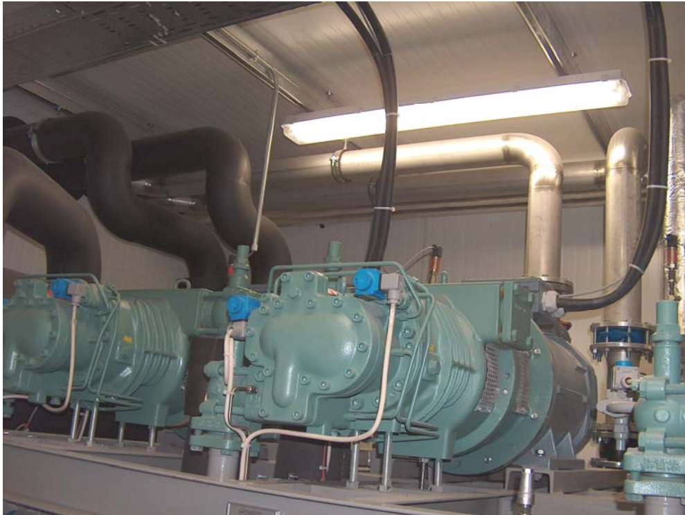
Rack com compressores Octagon (CO2)
